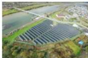
"Asahikawa Hokuto Solar Power Plant," a 1.25MW solar plant using bifacial solar panels (source: Nishiyama Sakata Denki)
